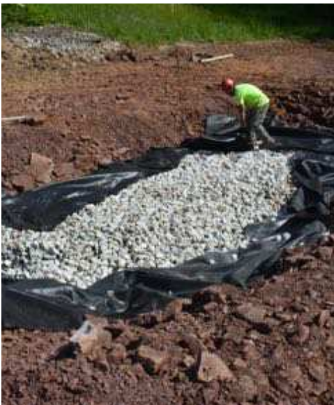
Construction of settling pool
