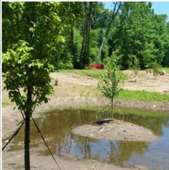
Construction and planting of forebay
