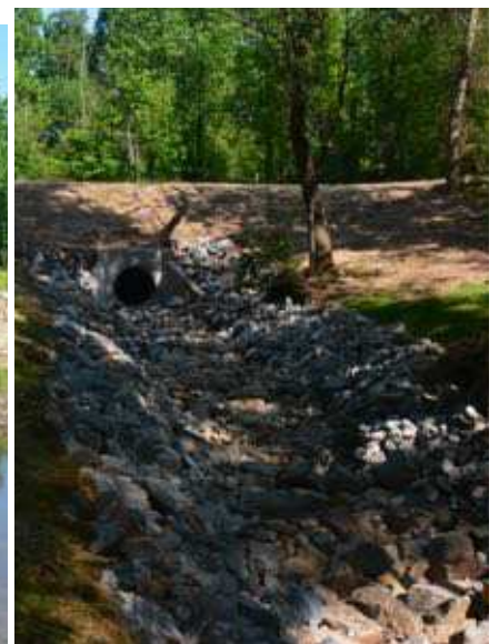
Restoration of streambank at outfall
