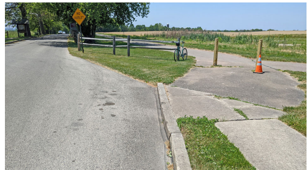
6" high concrete curb blocks the connection between the Upper Farm Road side path and Barley Sheaf Drive. This curb should be removed and replaced with an ADA-compliant curb cut
