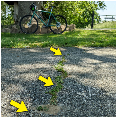
Tree roots erupting through the asphalt trail surface pose a potential hazard
