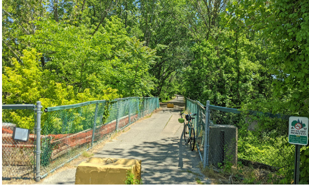
Hospital Bridge carries Lower Farm Road over Stony Creek. Concrete deterioration has necessitated the placement of fences restricting access to one half of the bridge deck
