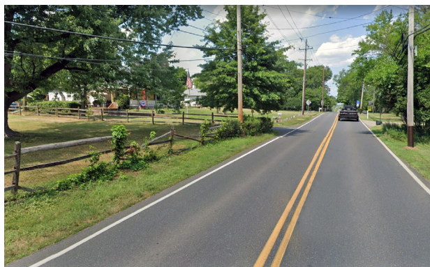
Two stretches of North Wales Road in Upper Gwynedd Township are only 22 feet wide with no sidewalks. One stretch does not have, and the other may have, sufficient right-of-way for a trail
