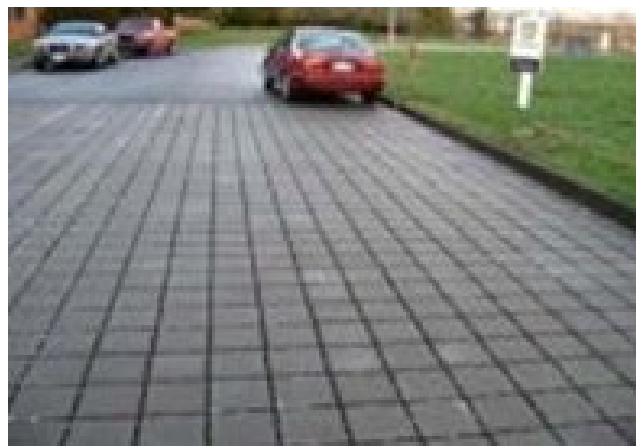
Figure 3. Permeable Pavement Example (EPA)
