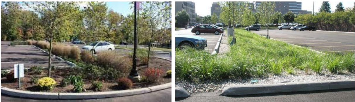
Figure 5. Typical buffer vs. enhanced stormwater management function (MCPC Parking Guide)
