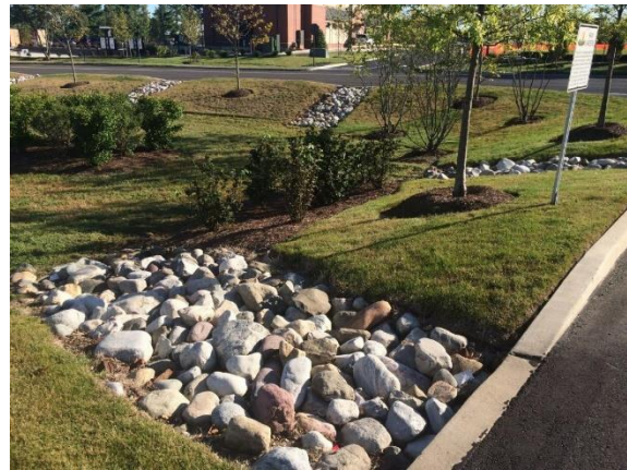
Figure 7. Rain Garden Features - Wegman's Parking Lot, Montgomeryville PA (PEC)
