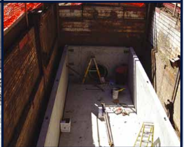
Subsurface system under construction
