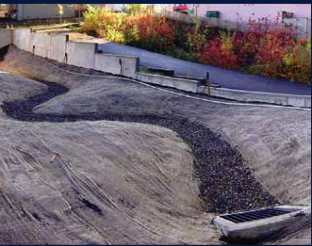
Meandering swale under construction
