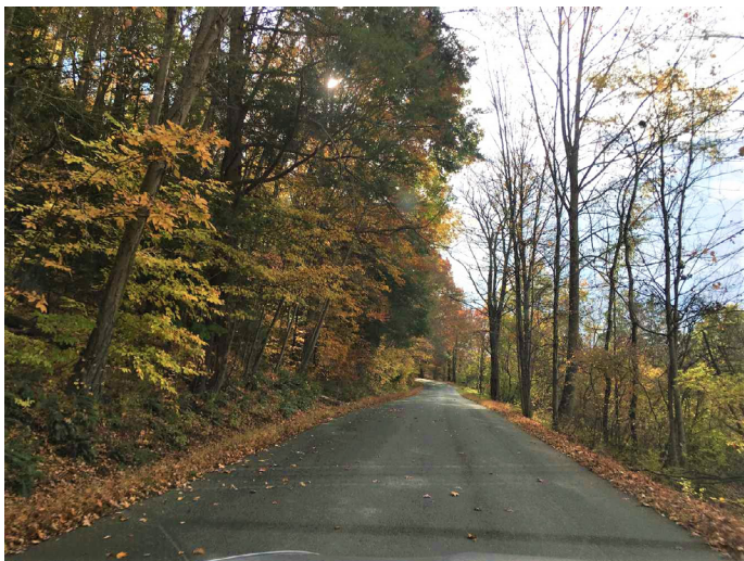
Figure 7: Haney Road typical conditions.
