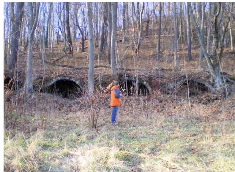
(B) Typical condition of most of the bank of 60 ovens, where 50 percent or more of the crown remains on each oven.
