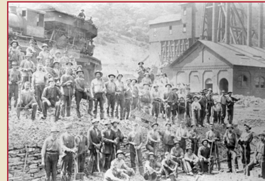
In this 1899 photograph, you can see the wooden coal tippie behind the coke workers. Men used the fourteen-tine coke forks to transfer the steaming coke into wheelbarrows which were then dumped into waiting railroad cars for the trip to the blast furnaces.
