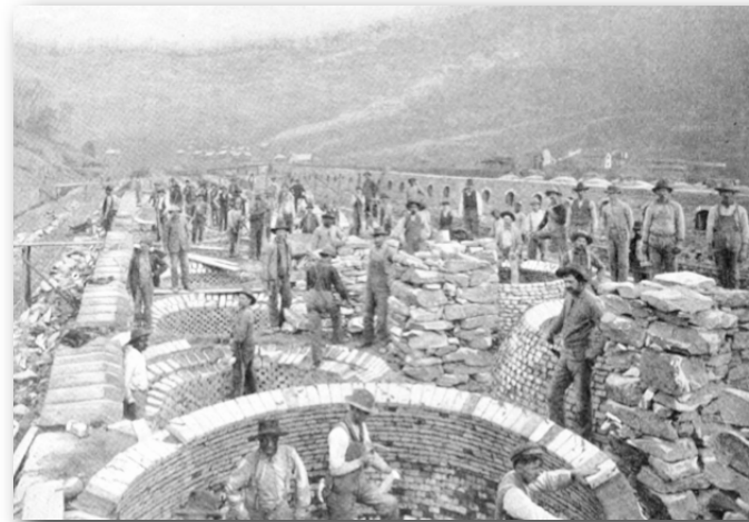
LABOR—Constructing beehive coke ovens.
