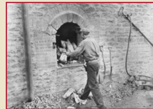
From atop, lorry wagons emptied coal into the hot ovens. The front openings were bricked up to control the burn. Two or three days later, the finished coke was pulled out. By 1910, 44,252 of the 55,166 coke ovens in Pennsylvania were located in the Connellsville Coke Region.
