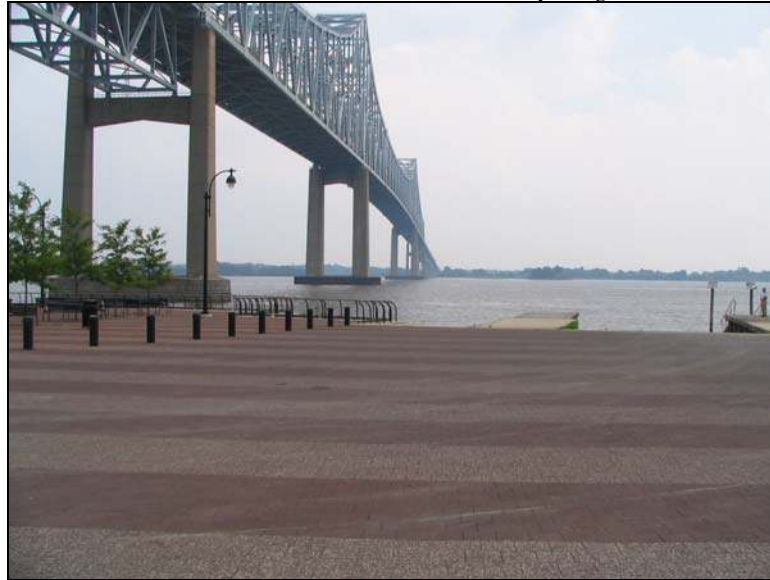
Delaware River at the Commodore Barry Bridge
