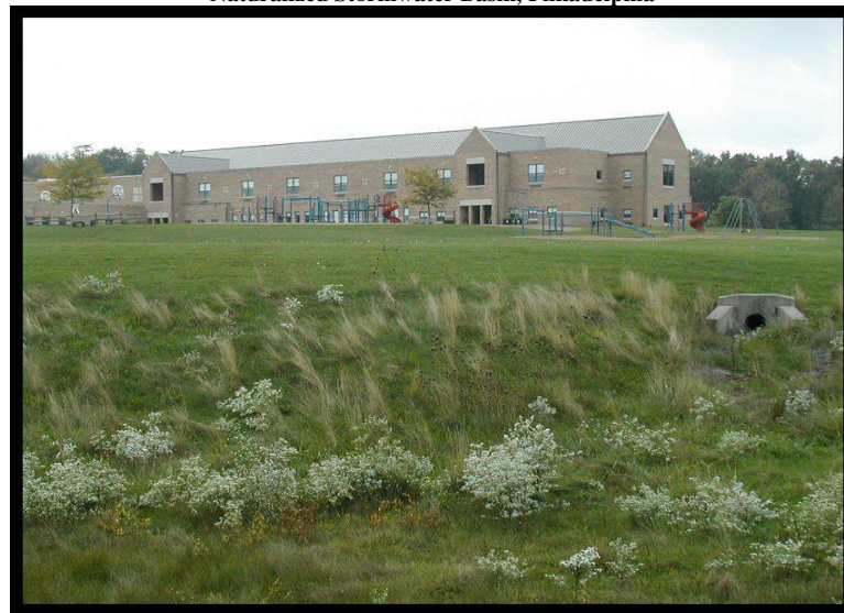
Naturalized Stormwater Basin, Philadelphia
