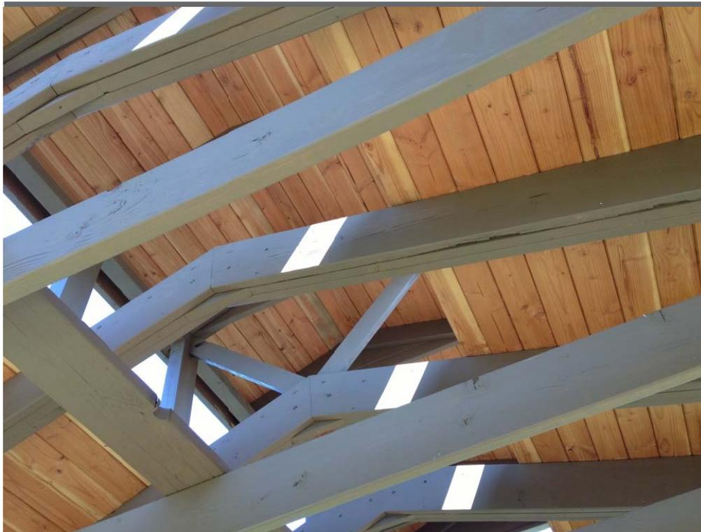
*A view of the roof interior showing structural framing and cupola. The tongue and groove wooden planks will demonstrate that the green roof does not leak.*
